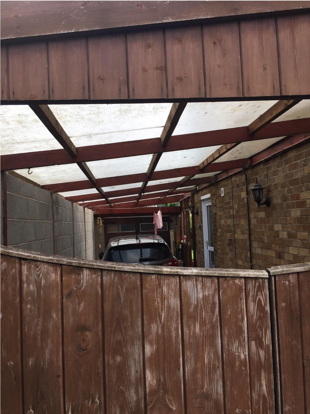
Views through the car port towards the applicant's garage
